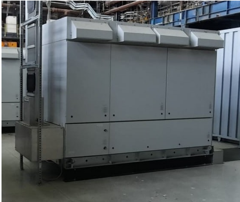
Figure 40: External IP 55 for the PCS system
